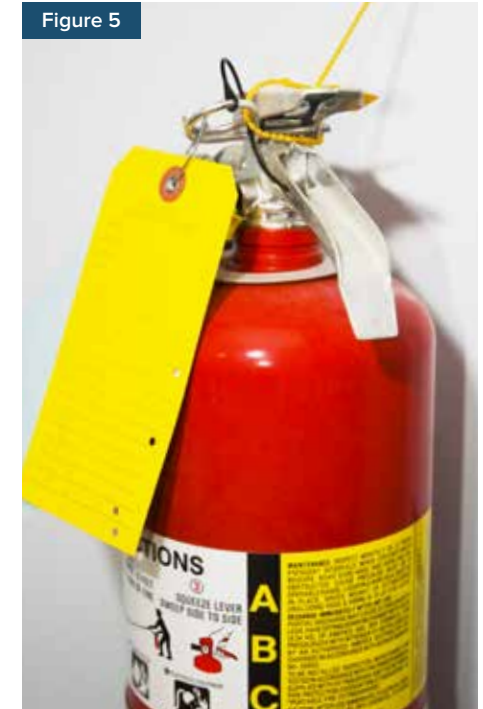
Fire Extinguisher with Inspection Log
