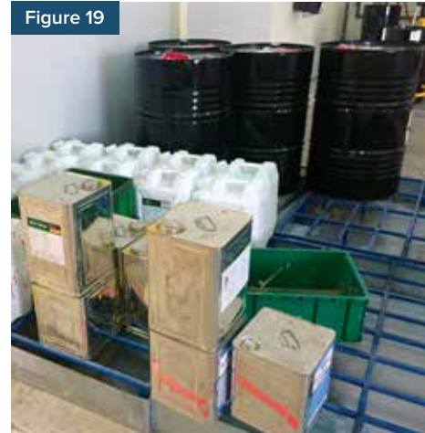
Chemical storage room with secondary containment device
